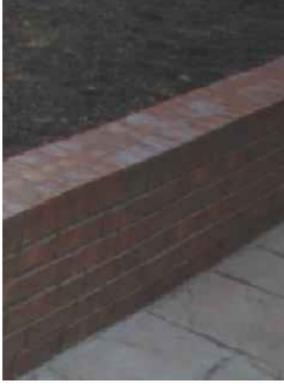
C) Typical example of Brick retaining wall
