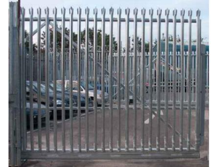
G) Single Palisade gate to Allotments. 3.0m metres wide, finish to be powder coat Green
