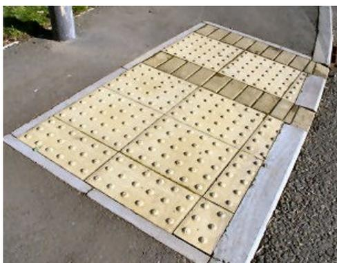
**Raised table ramp** – raising the road surface (usually of a side road) at a junction so that it’s the same height as the pavement, so that vehicles on the road slow down and pedestrians have priority. Example below:
